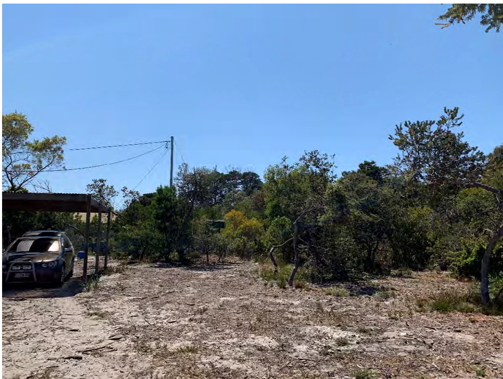
Clearing around existing carport to be demolished
