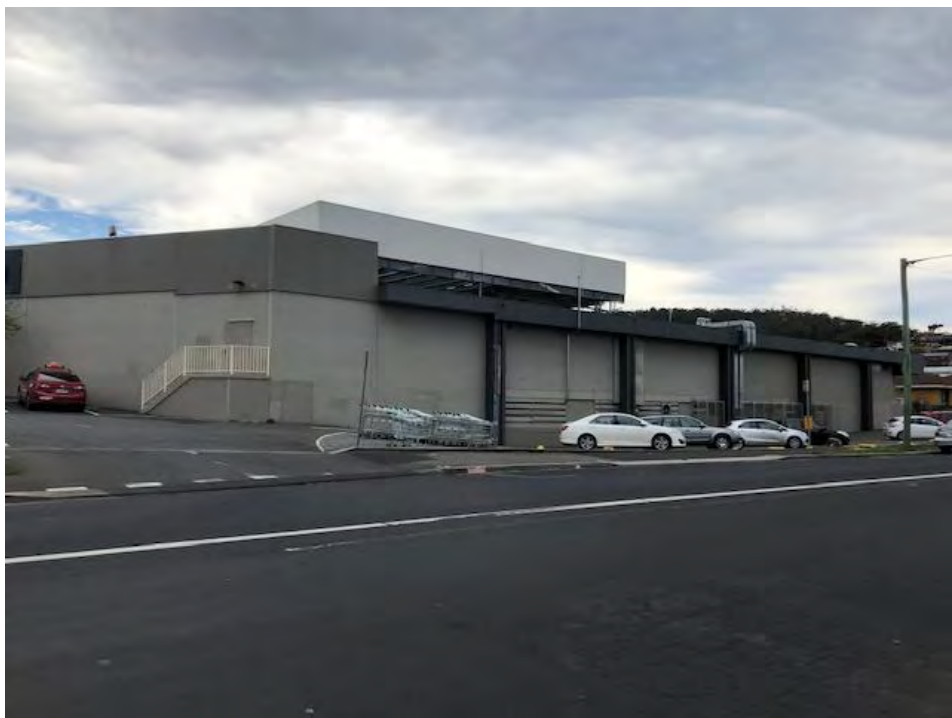
View of the site from Clarence Street looking north east.
