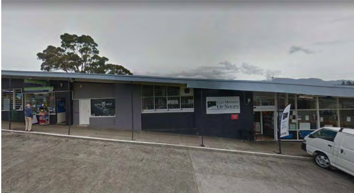
Existing City Mission Shop (Shop 5) viewed from Edgeworth Street.
