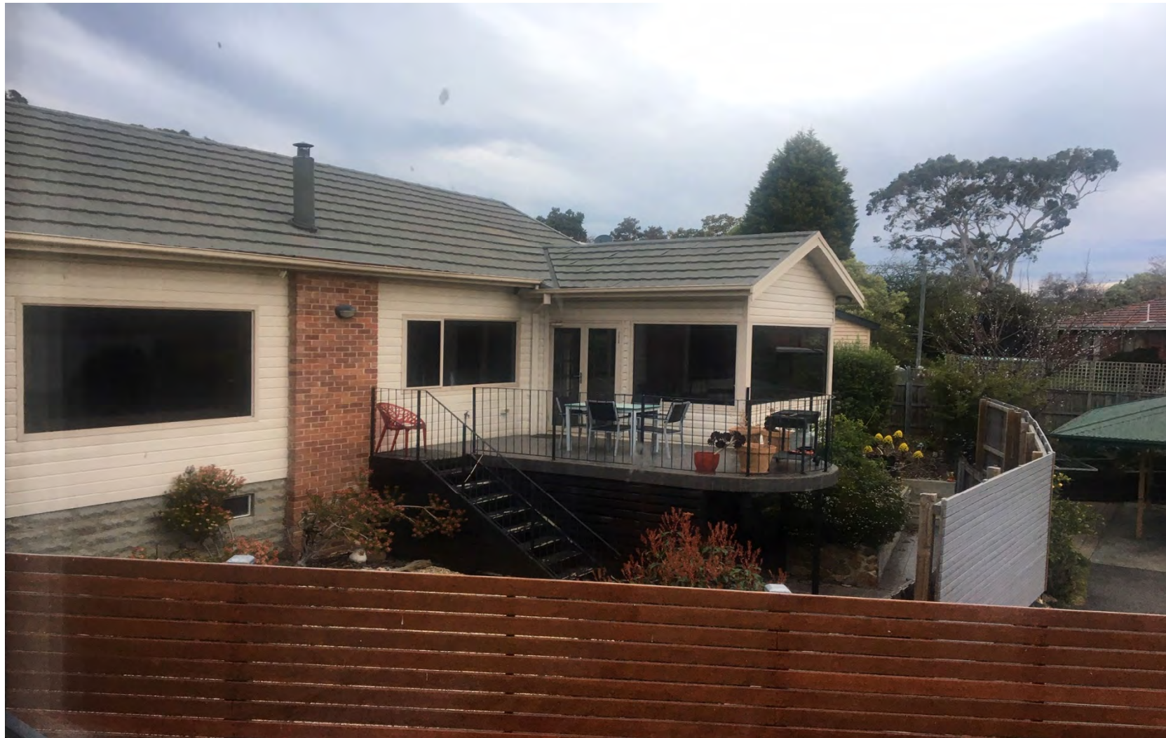
Photo 2: Site viewed from northern property boundary
