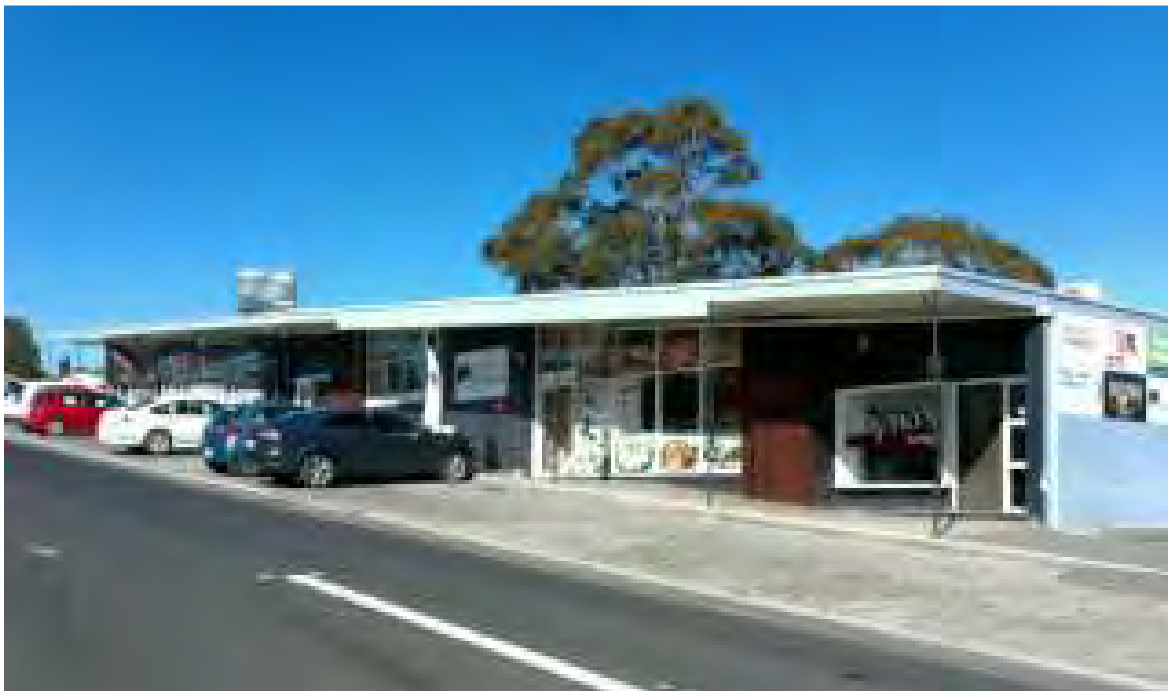
Commercial building showing existing 7 tenancies viewed from Edgeworth Street.
