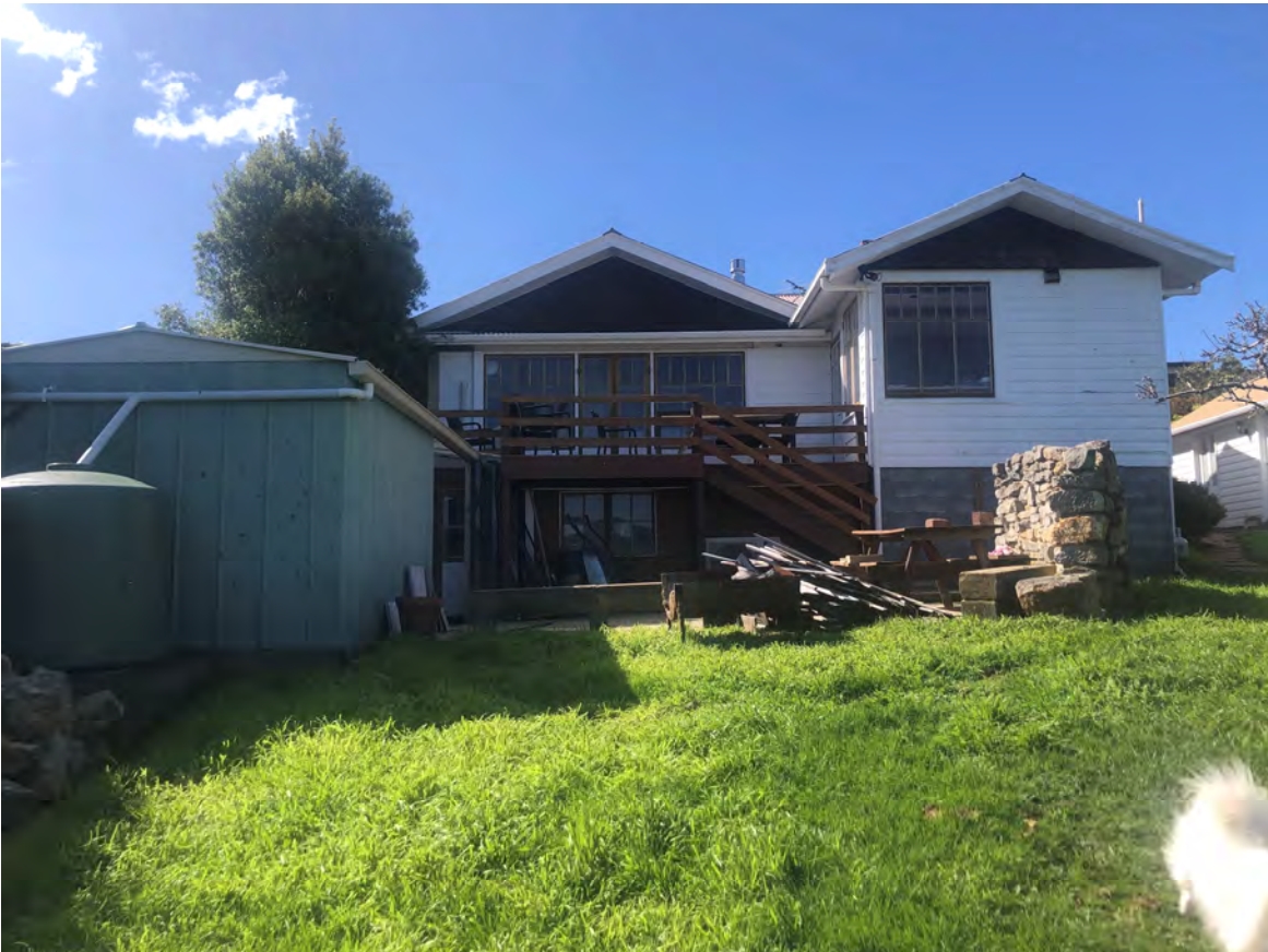
Photo 2: Site viewed from adjacent southwestern boundary, looking northeast.
