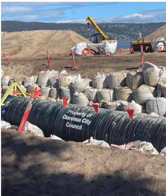
■ Beach Street stormwater upgrade, Bellerive.
