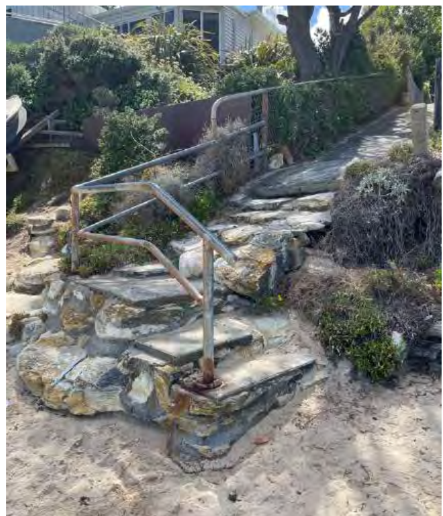
Existing stairs to beach
