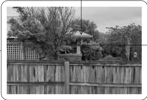
existing habitable room window
