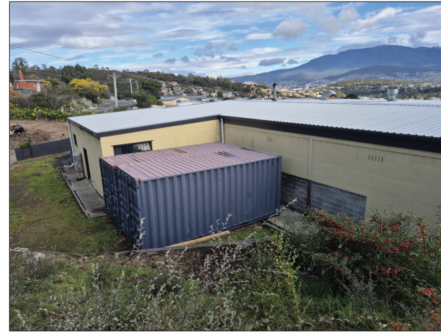
STORAGE CONTAINERS # 7 - 8 NORTH EAST VIEW
