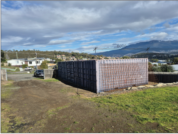
STORAGE CONTAINERS #1 - 5 NORTH EAST VIEW
