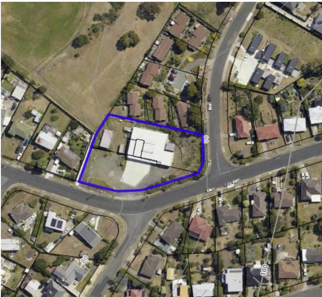
Figure 1: Aerial image of the Site (Source: List Map)
