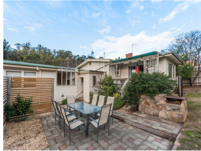
EXISTING BACK VIEW
