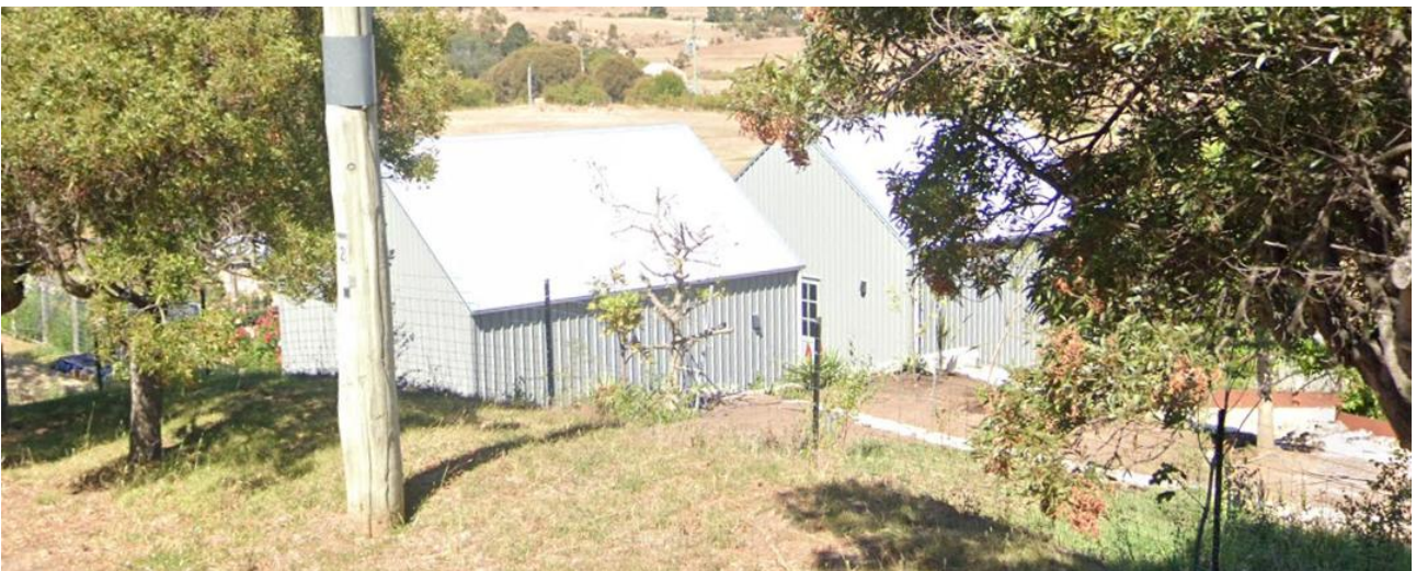
Figure 3: The two outbuildings.
