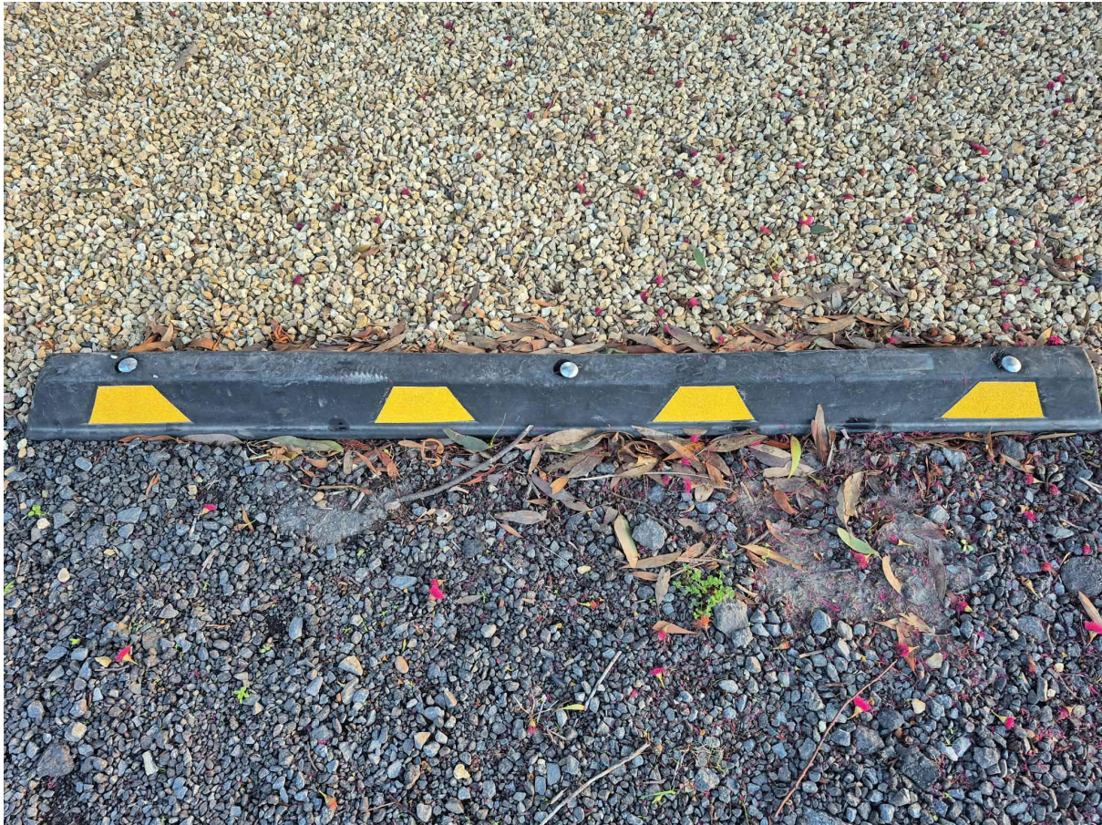
Photo 2 – Existing pinned bollard/wheel stop
