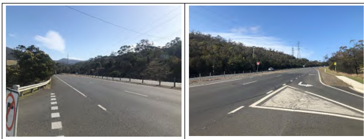
Figure 2 East Derwent Highway
