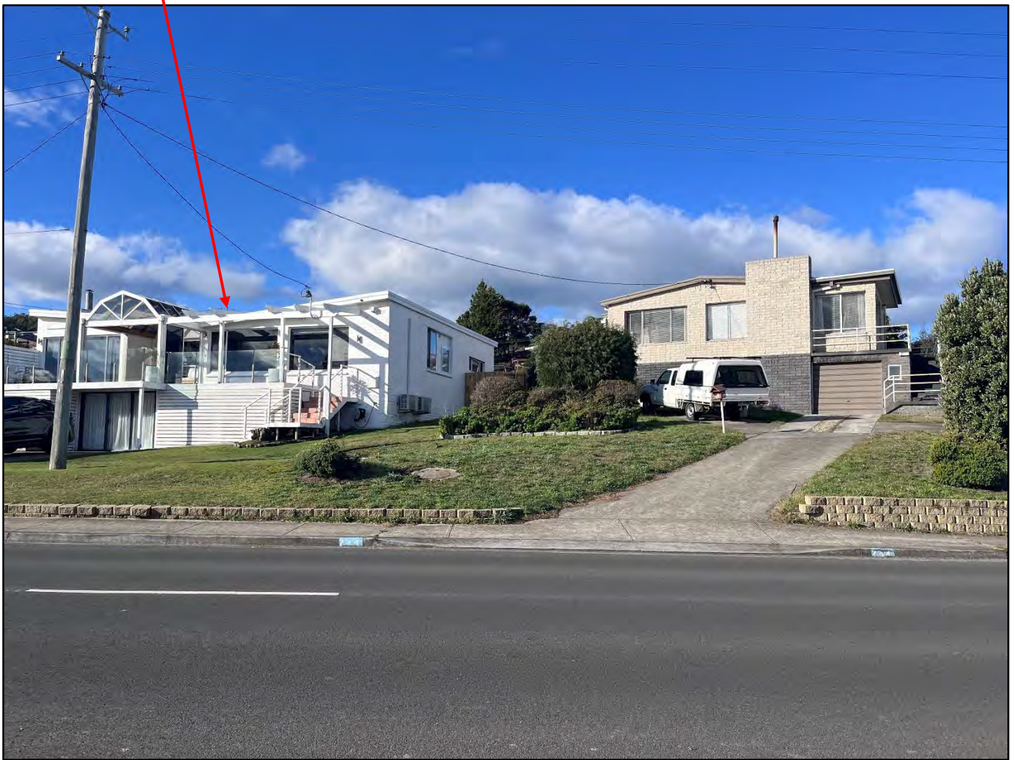
Fig.1 – View from Tranmere Road of the subject site and the adjoining property at 244 Tranmere Road, Tranmere
