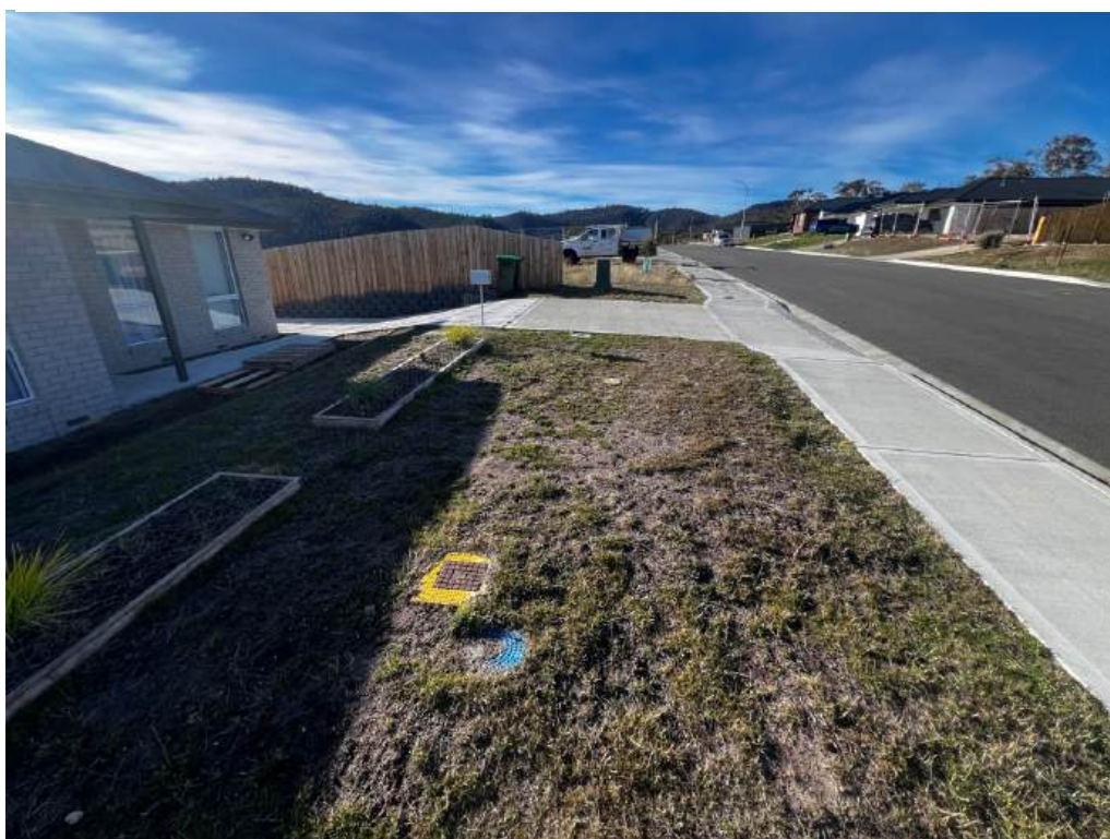
Image 8: Existing fire hydrant along Bottlebrush Way (Photo taken on site 22/5/2026)
