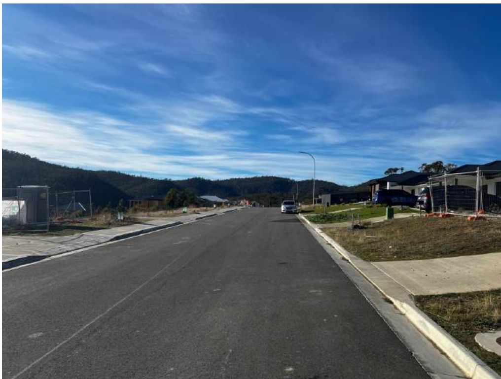
Image 11: Bottlebrush Way, looking East (Photo taken on site 22/5/2026)
