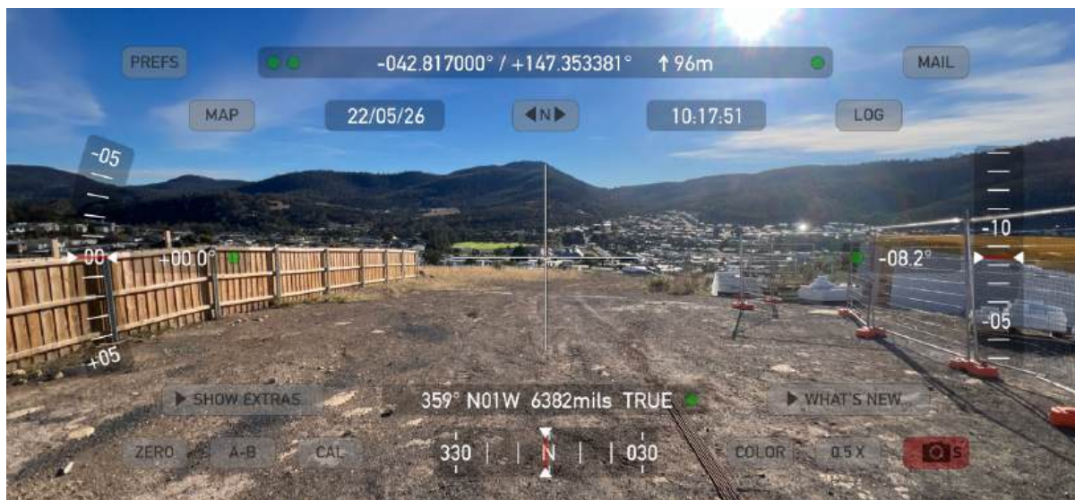
Image 3: Northern Azimuth (Photo taken on site 22/5/2026)
