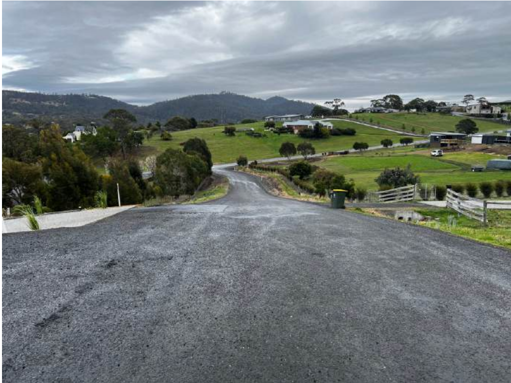
Image 11: Eleanor Court, looking West (Photo taken on site 26/9/2025)
