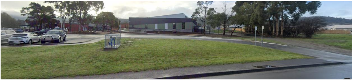
Figure 14: The sealed exit from the church carpark (Google Street View)
