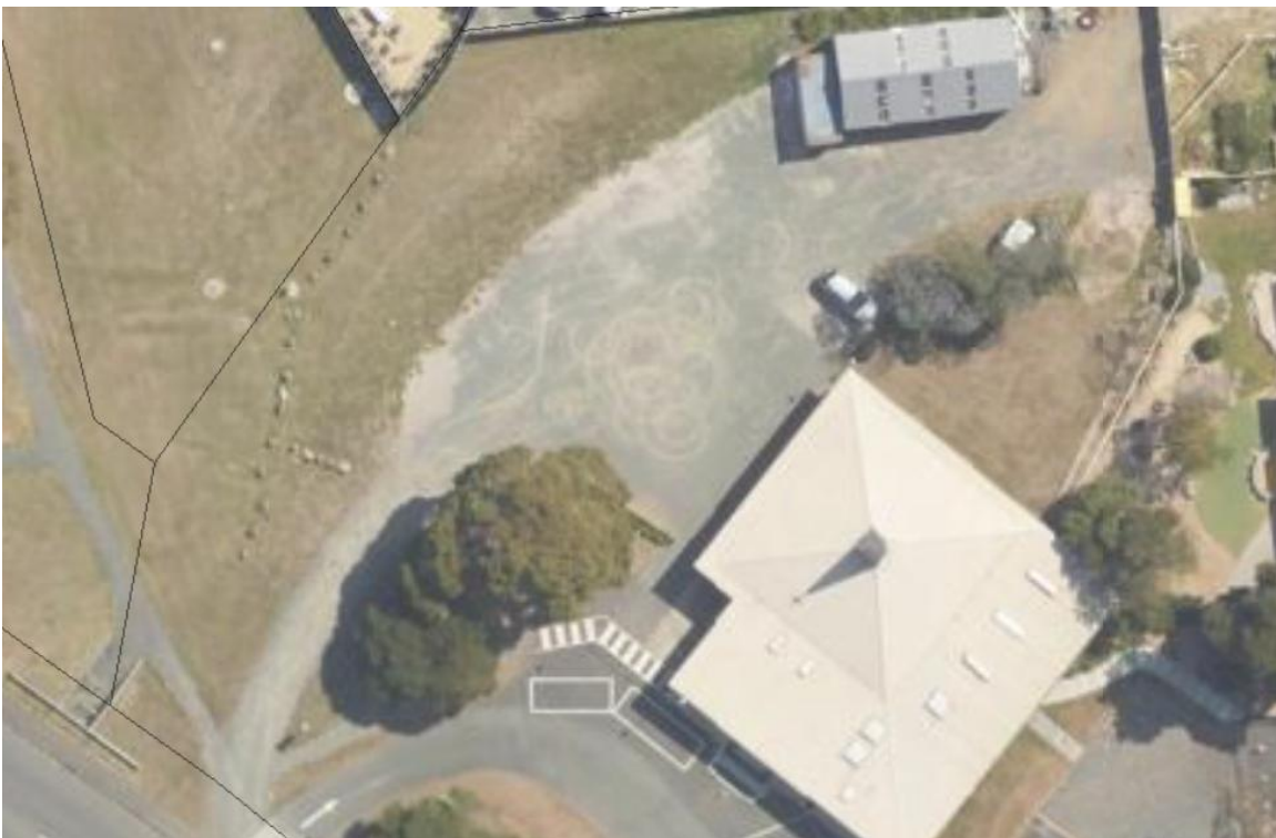
Figure 12: The gravel staff carparking area providing for at least 17 vehicles (LIST State Aerial Photo).
