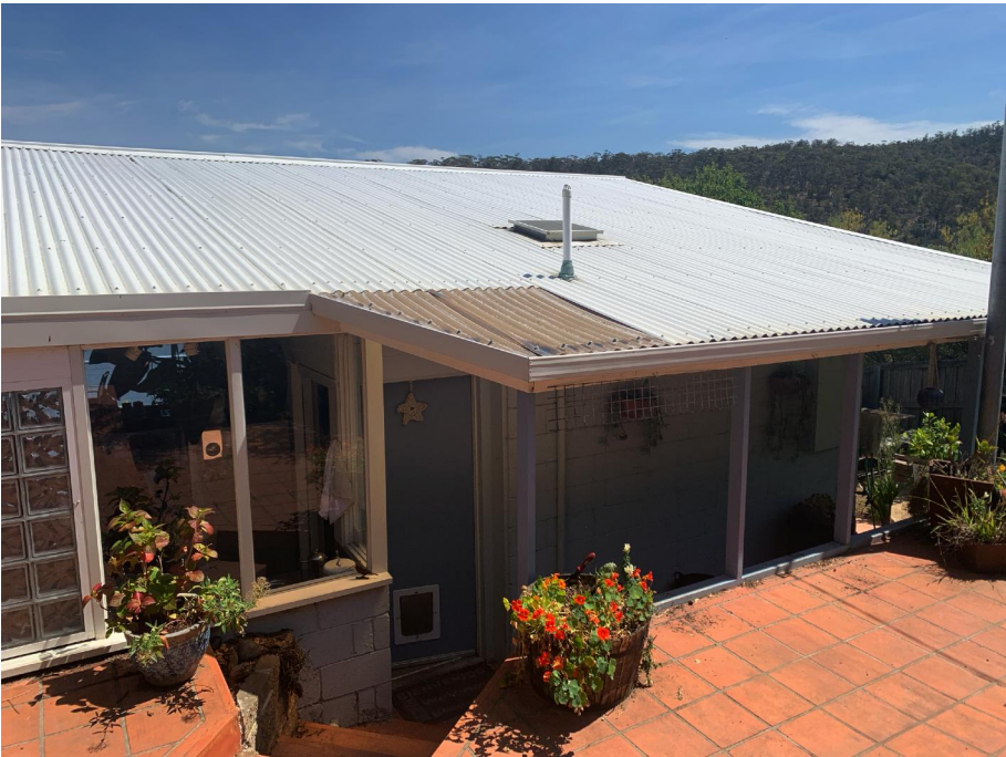
REAR ENTRY AND PAVING
