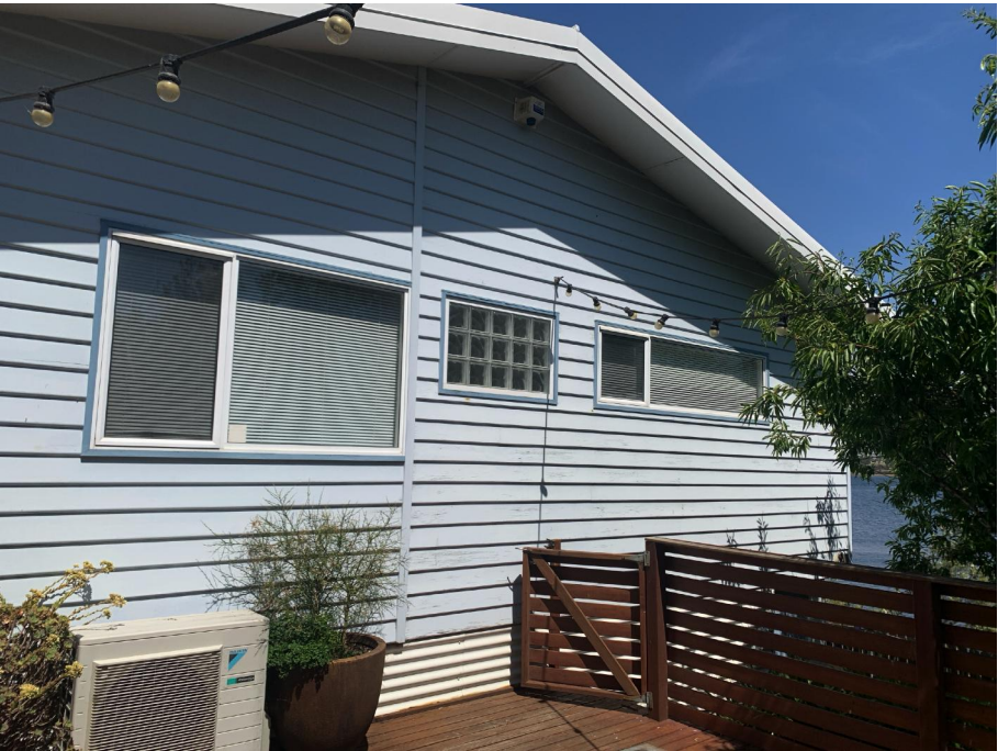
EAST ELEVATION AND SIDE DECK
